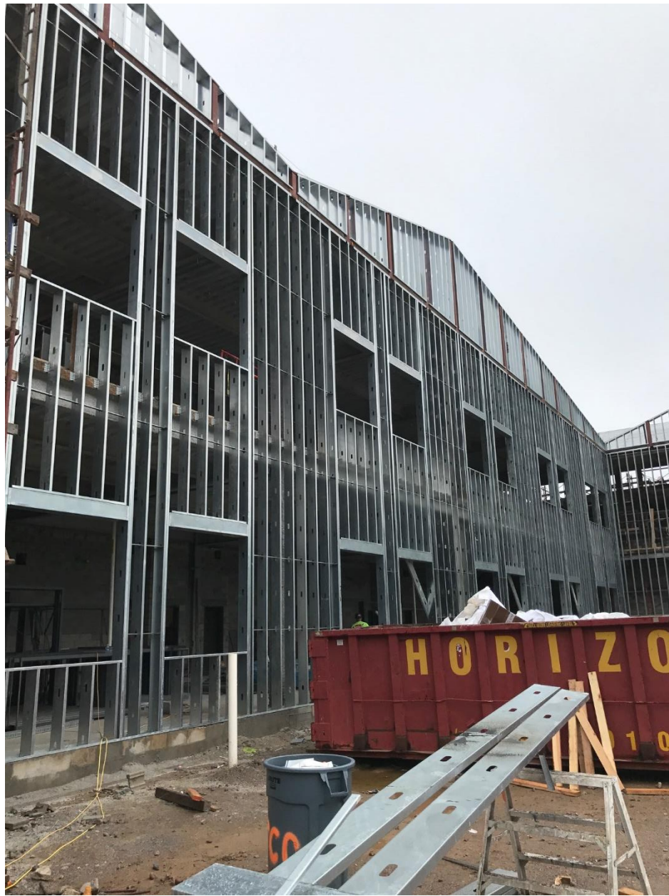
Trenton Central High School under Construction
